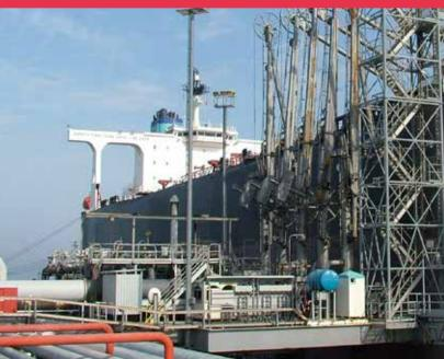
In the last step, the crude oil is loaded into the tankers through loading arms installed on the export berths.
